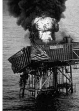
Ignition of flammable materials causes catastrophic results.
