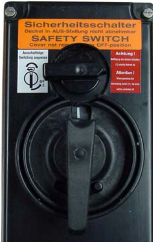
The control circuit top switch must be turned off before breaking the main supply on the SpecOne™ Zone 1 VFD switch.
