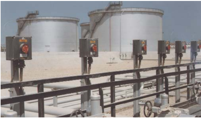
The Cooper Crouse-Hinds GHG 26 Series, nonmetallic 10 to 180 amp motor disconnect switches are rated IP 66 and are UV protected for extreme outdoor environments
