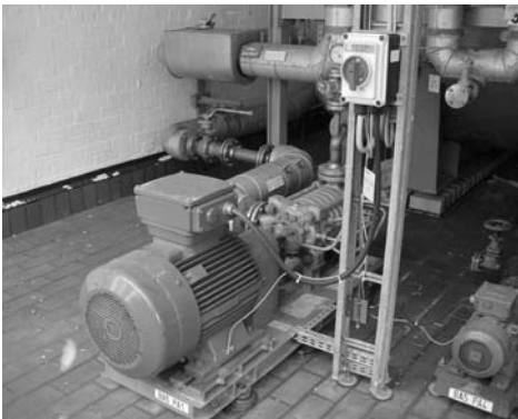
The Cooper Crouse-Hinds GHG 26 Series, nonmetallic 10 to 180 amp motor disconnect switches are rated IP 66 and are UV protected for extreme outdoor environments
