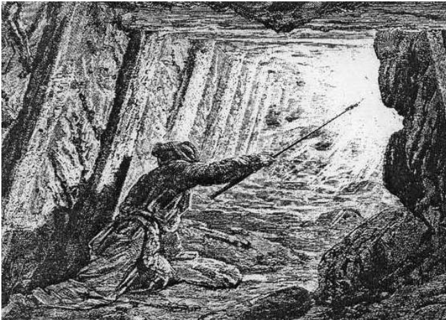
Igniting small pockets of methane gas was one of the original methods to prevent ignition in coal mines
